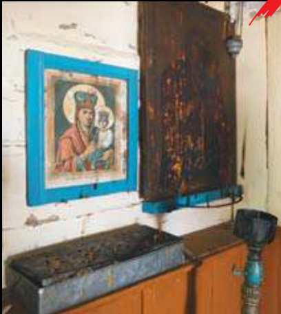
Candle stand placed under the icon and in the proximity of the wooden wall. Placement of candles can also cause a fire.
