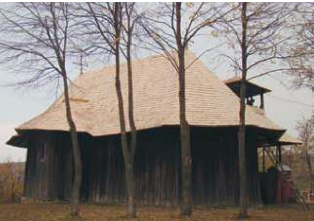
The church after repairs and replacement of zinc steel roofing with wooden shingles.
