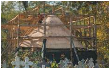
Rebuilding the wooden shingle roofing, 2015.
