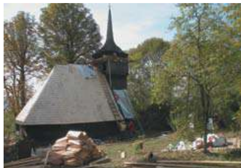
Image from shingle replacement process.
