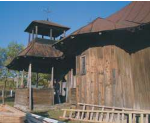
The church before repairs.
