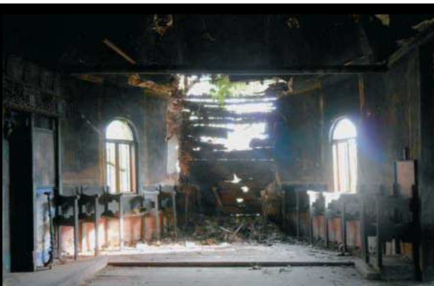
Serious degradation of the log wall caused by rain water infiltrated through the deteriorated roof.
